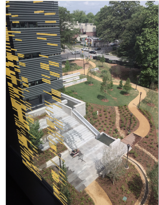
The Engineered Biosystems Building has a window motif that resembles a radioactively labeled sequencing gel
